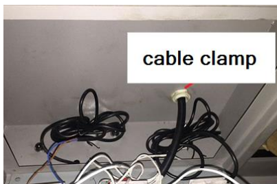
4. Cable clamp: Fix the control line with the cable clamp. Replace and fix the control panel cover!
